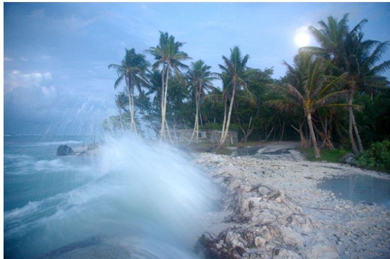
Waves crashing over roadway in Temwaiku, Kiribati. Courtesy of Annika Dean.
